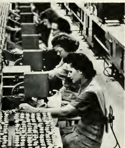
Electron guns are assembled here and microscopically tested to watch-makers' rigid specifications.
