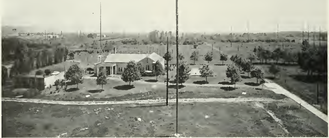
NBC's East Coast transmitter building at Bound Brook, N. J., is surrounded by a forest of poles supporting the station's array of shortwave antennas.
