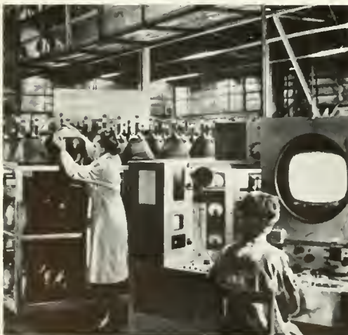
As a tube approaches completion it is tested for picture brightness under home lighting conditions.
